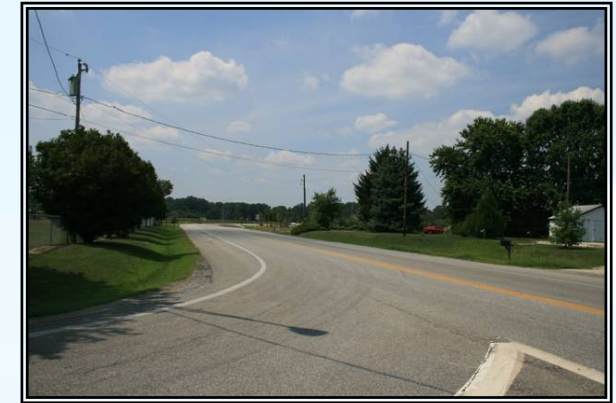
Intersection of Main and Rte 300 looking west
